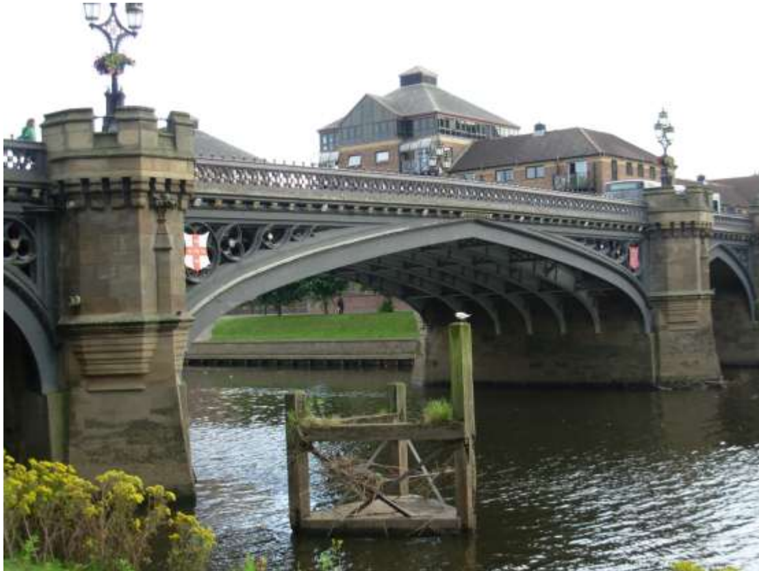
Skeldergate 1878: The bridge is essentially an iron structure, it was clad in stone and given mediaeval details, such as the turrets, to emphasise its solidarity. Note the heraldic details; the city arms and the arms of the archbishopric flank the arch.
