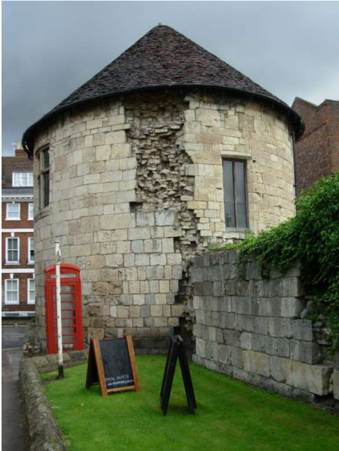
St Mary's Tower, showing the join where it was reconstructed to a narrower diameter after destruction in the Civil War.
